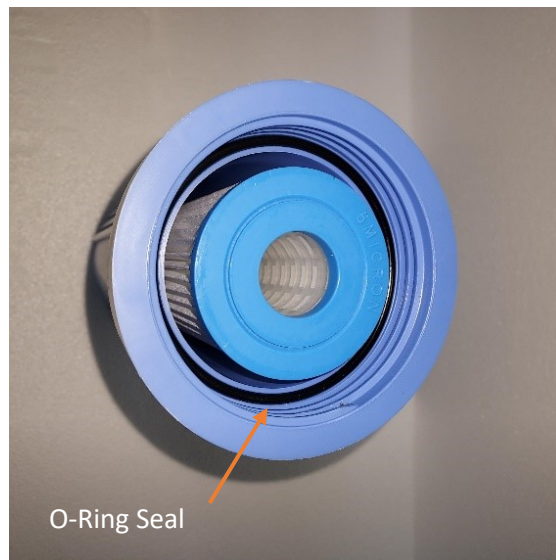
Figure 25: 5 Micron Pre-Filter
