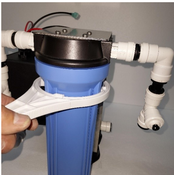
Figure 25: 5 Micron Pre-Filter
